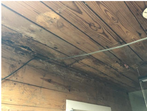
Termite Damage
