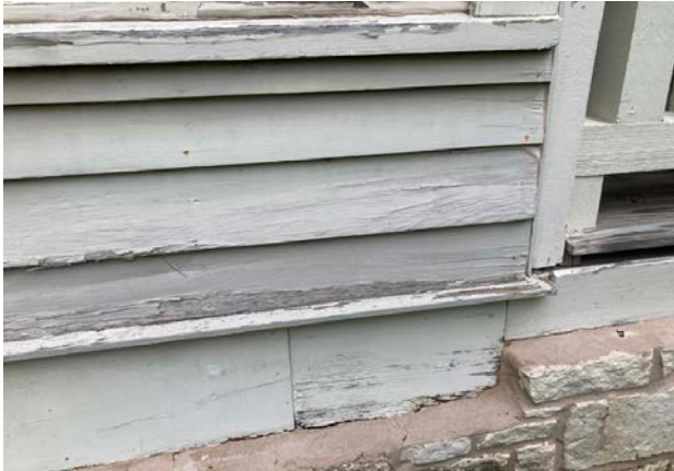
Current conditions of wood siding
