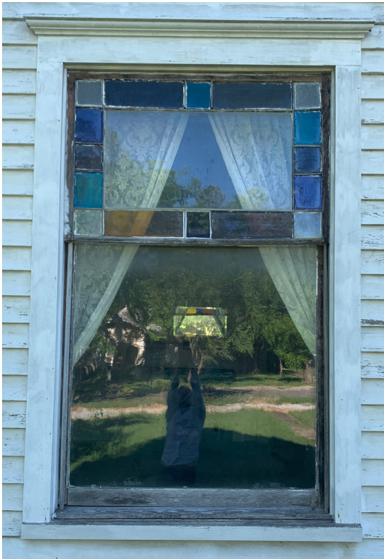
Existing stained glass windows to be refurbished
