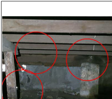
View of pier and beam foundation Wooden supports in contact with earth
