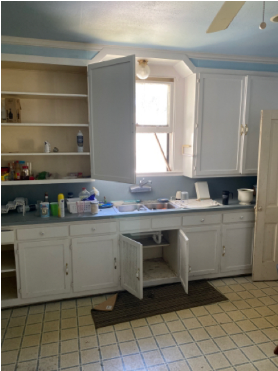
Kitchen cabinets appear water damaged underneath the sink
