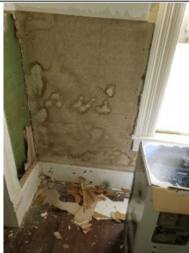
Water damage Mildew
