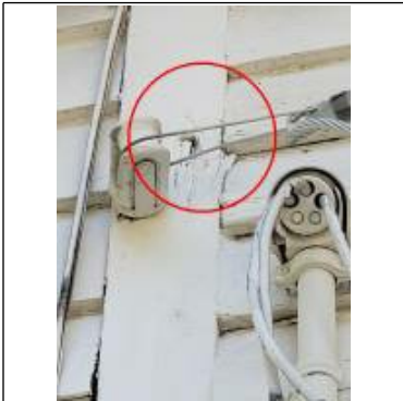
Wood deterioration
