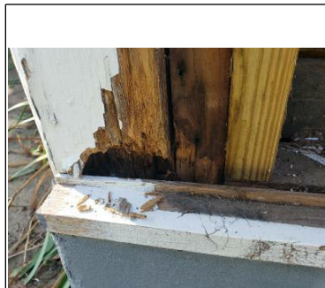
Weird deterioration/rot noted
