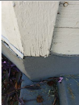
Wood deterioration noted
