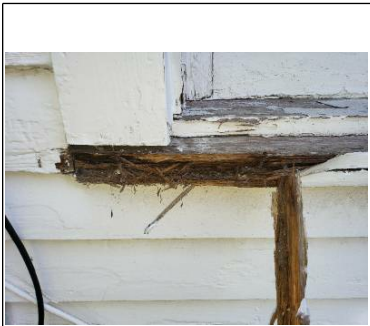
Wood rot/deterioration
