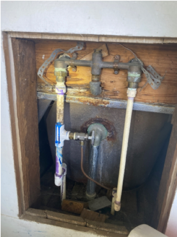
Water damage to the framing, this is the hall bathroom next to the kitchen and porch.
