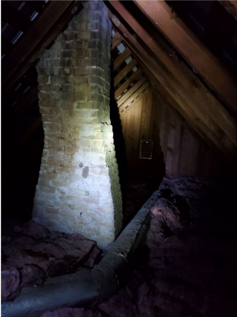
Photo #24, Chimney in attic of 1890s home. Note minimal bracing. Chimney is no longer in service due to leakage and old mortar. We plan to remove it and replace it with an externally similar chimney.
