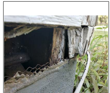
Wood deterioration/rot noted
