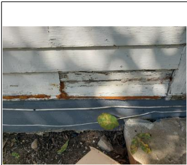
Wood deterioration/rot Expanding foam
