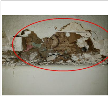
Wood deterioration Water staining Possible mildew
