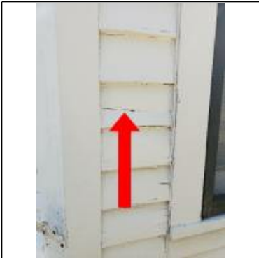
Damaged/ cracked siding
