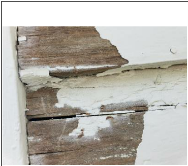
Wood deterioration noted
