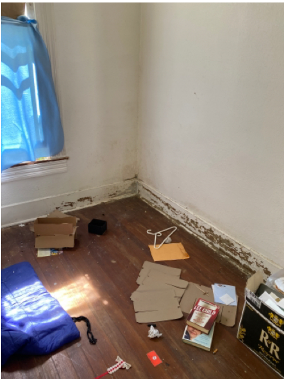
Baseboards are water damaged with visible growth.
