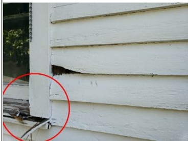
Damage noted Wood deterioration/rot
