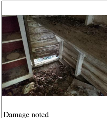
Wood deterioration/rot
