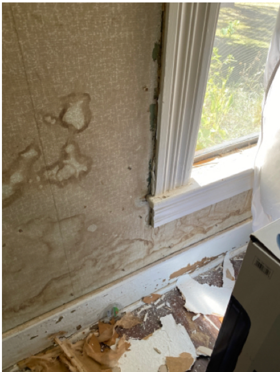
Water damage around the windows in the home.
