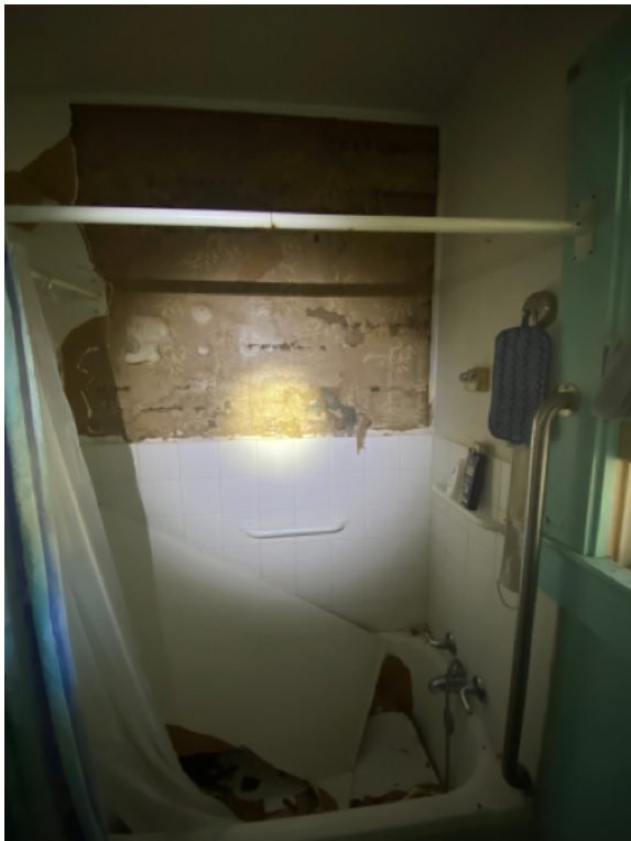
Water damage and apparent growth in the wall in the bathroom.
