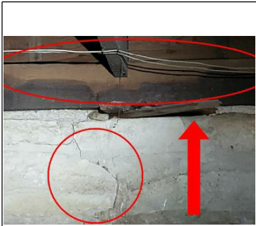
Inadequate shims noted Cracking noted Heavy Moisture noted
