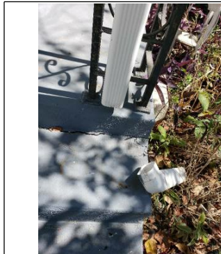
Damaged gutters
