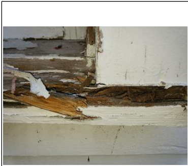
Wood deterioration noted
