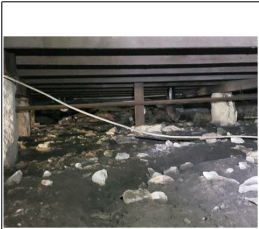
Pier and beam foundation view
