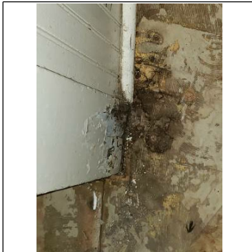
Water damage Fungal growth
