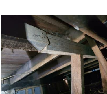
Damaged beams noted
