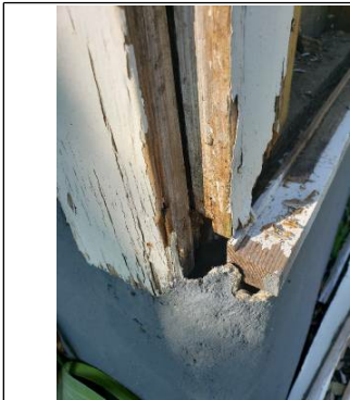
Wood deterioration/rot noted
