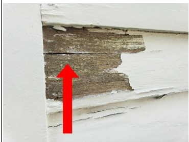
Damaged siding
