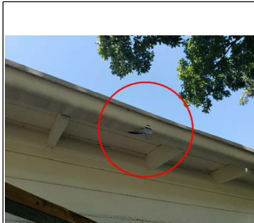
Damaged gutters
