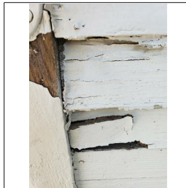
Wood deterioration noted
