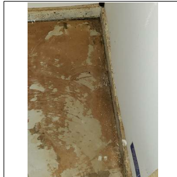
Water damage Fungal growth
