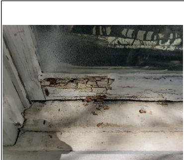
Wood deterioration/rot
