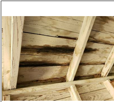
Wood deterioration/rot
