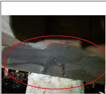
Wood deterioration noted Heavy moisture noted
