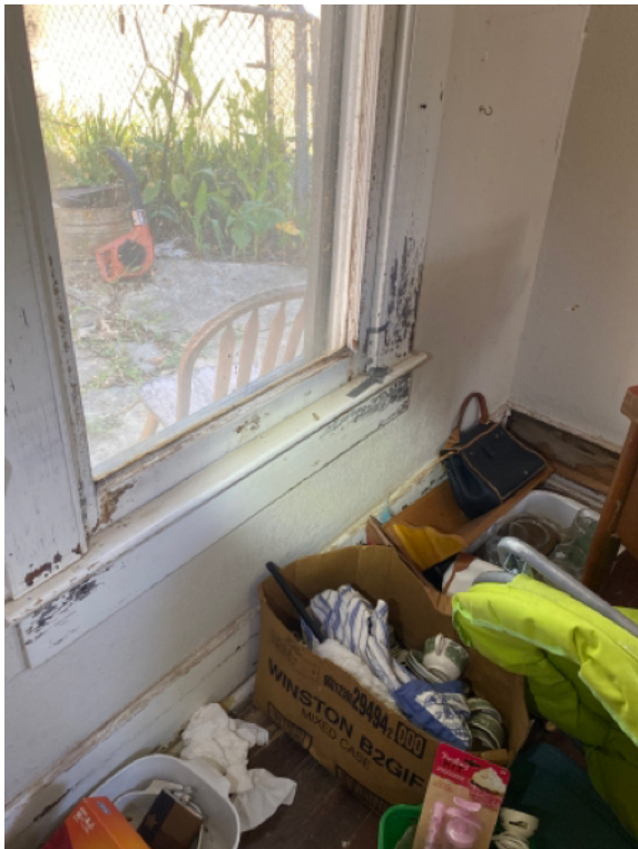
Water damage around the windowsills throughout much of the home.
