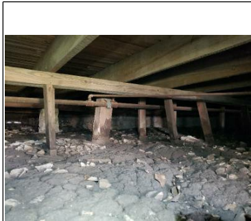
View of pier and beam foundation Wooden supports in contact with earth
