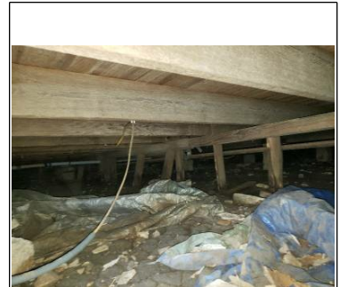
View of pier and beam foundation
