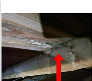
Wood deterioration noted
