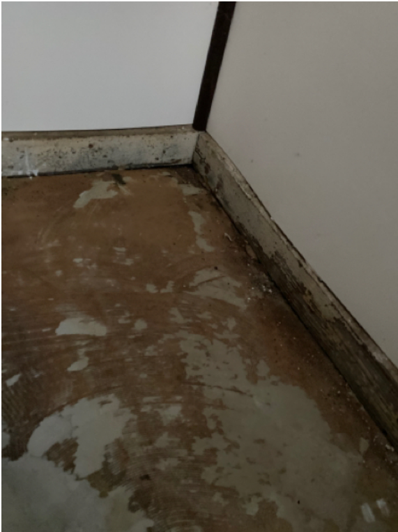
Kitchen pantry. Water damage and mold like growth at the base of the walls.
