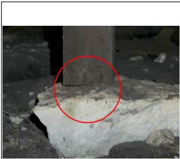
Wood deterioration noted
