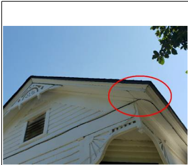
Wood deterioration
