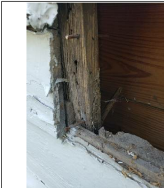
Wood deterioration noted
