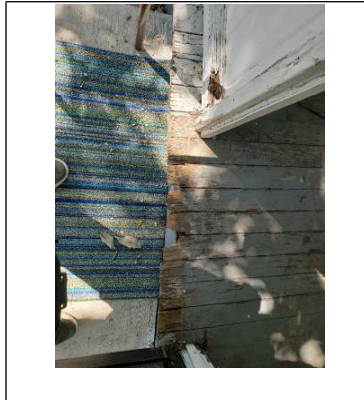
Wood deterioration/rot
