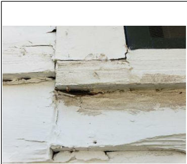
Wood deterioration
