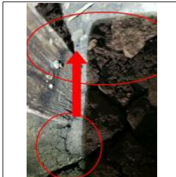
Wood deterioration noted
