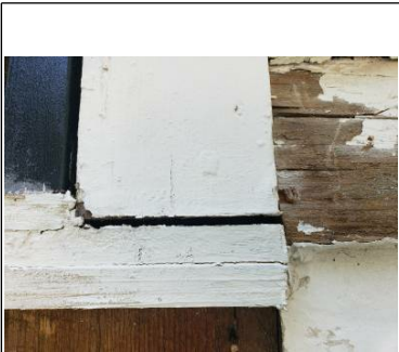
Window sill plate not securely attached
