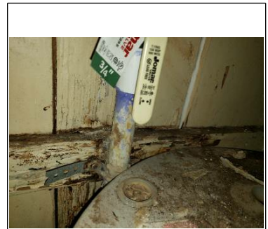
Wood rot Water heater closet
