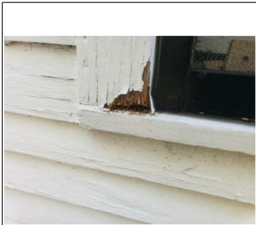
Wood deterioration
