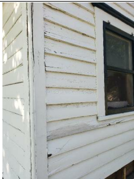
Wood deterioration/ water damage noted
