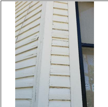
Wood deterioration noted
