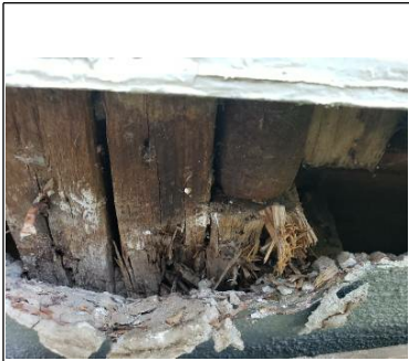
Wood deterioration/rot
