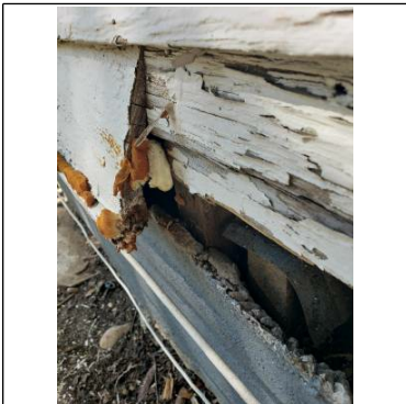
Wood deterioration/rot Expanding foam
