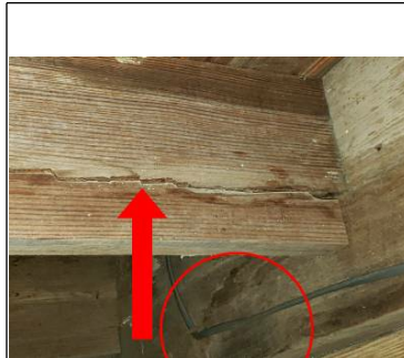
Water damage noted Cracking noted
