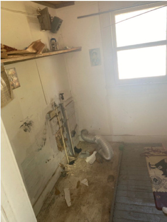
Water damage to the framing, this is the hall bathroom next to the kitchen and porch.
