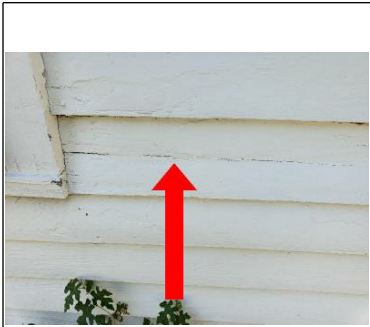
Cracked siding
