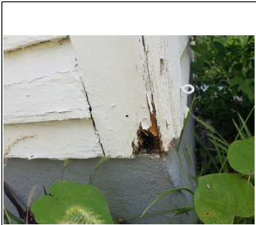
Wood deterioration/rot
