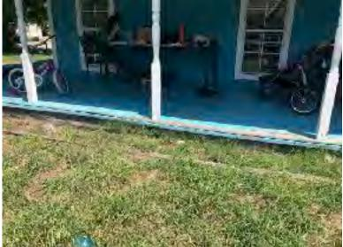
Condition of porches- dipping and severe splintering (left and below)
