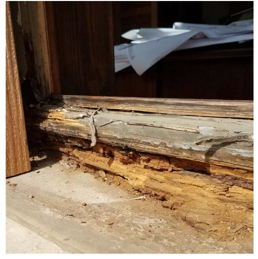
Example of water/moisture damage to wood window frame
