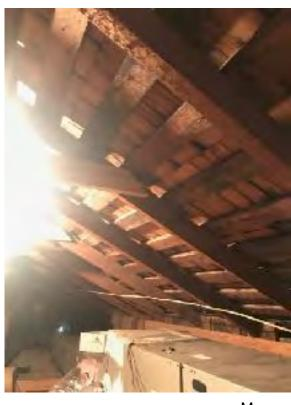
Current roof constructed over original roof (note shingles) causing original elevation to change (left)
