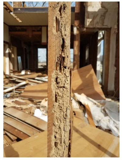
Example of termite damage to wood framing
