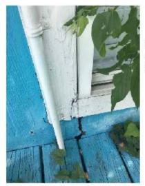
Crack in siding (left) Large tree root grew into home (right)
