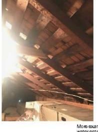
Current roof constructed over original roof (note shingles) causing original elevation to change (left)
