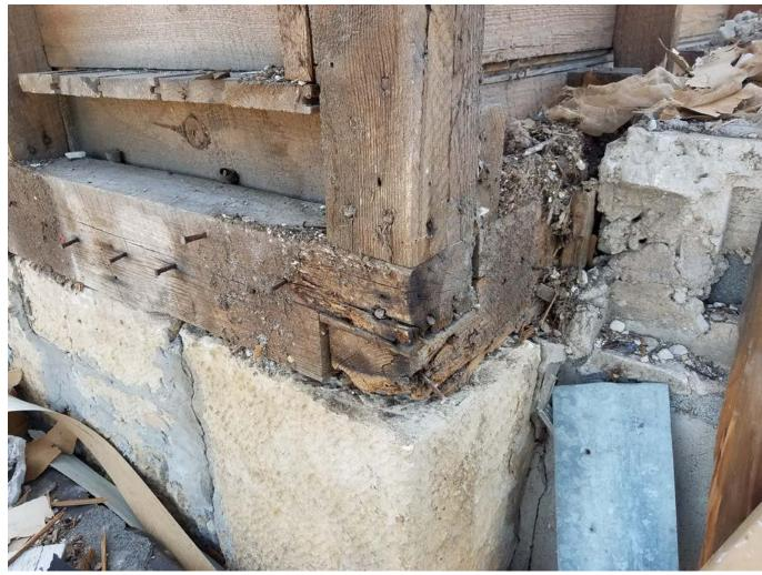
Example of water/moisture damage to wood floor beam and framing
