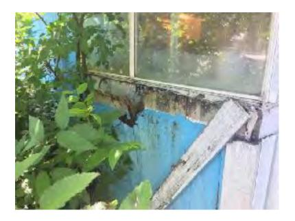
Insulation exposed where siding has decayed. (above and to left)
