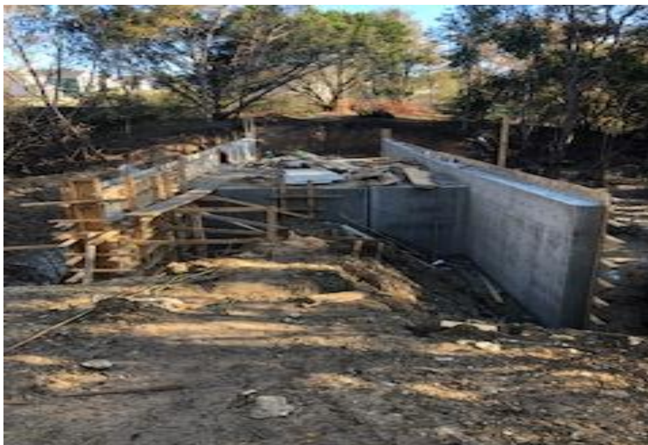
Box culvert installation
