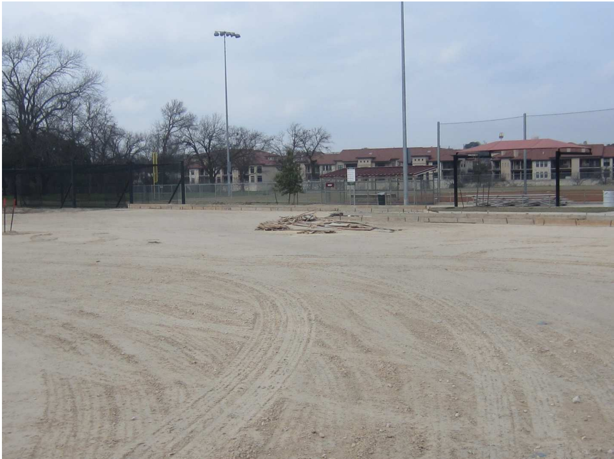
VFW Parking Lot Construction
