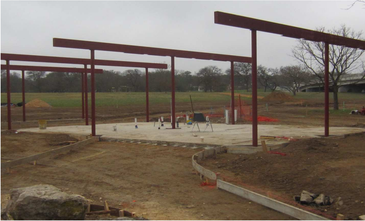
Restroom Frame Work
