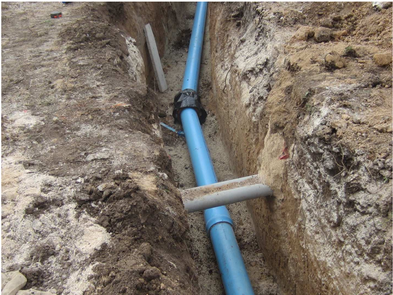
Water line installation
