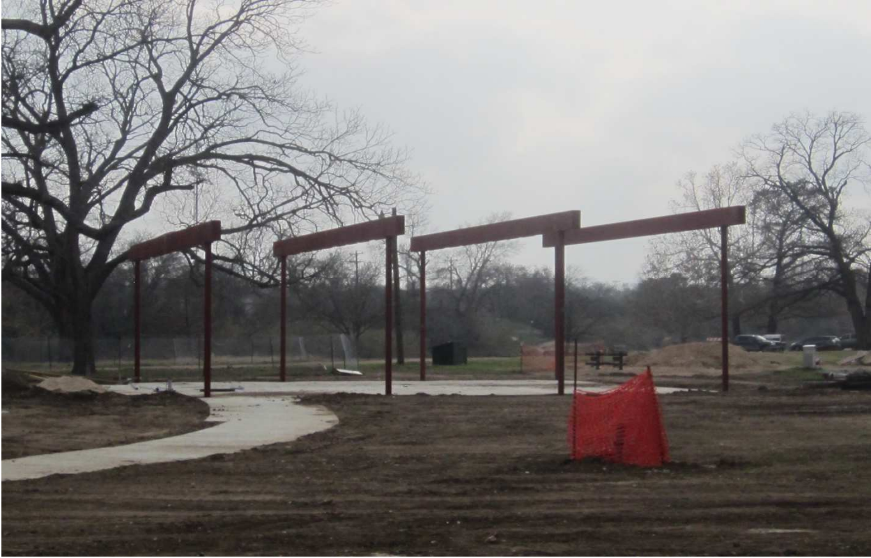
Large pavilion frame work
