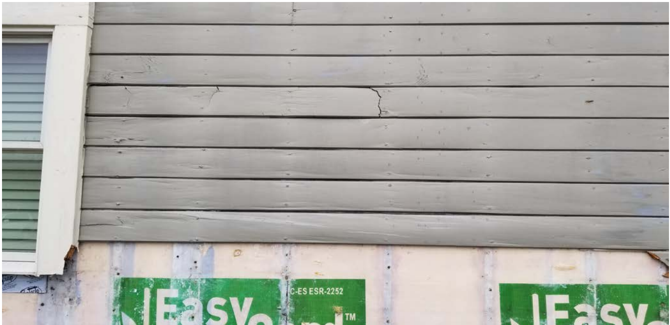
Picture 1: Deteriorated Siding and Trim
