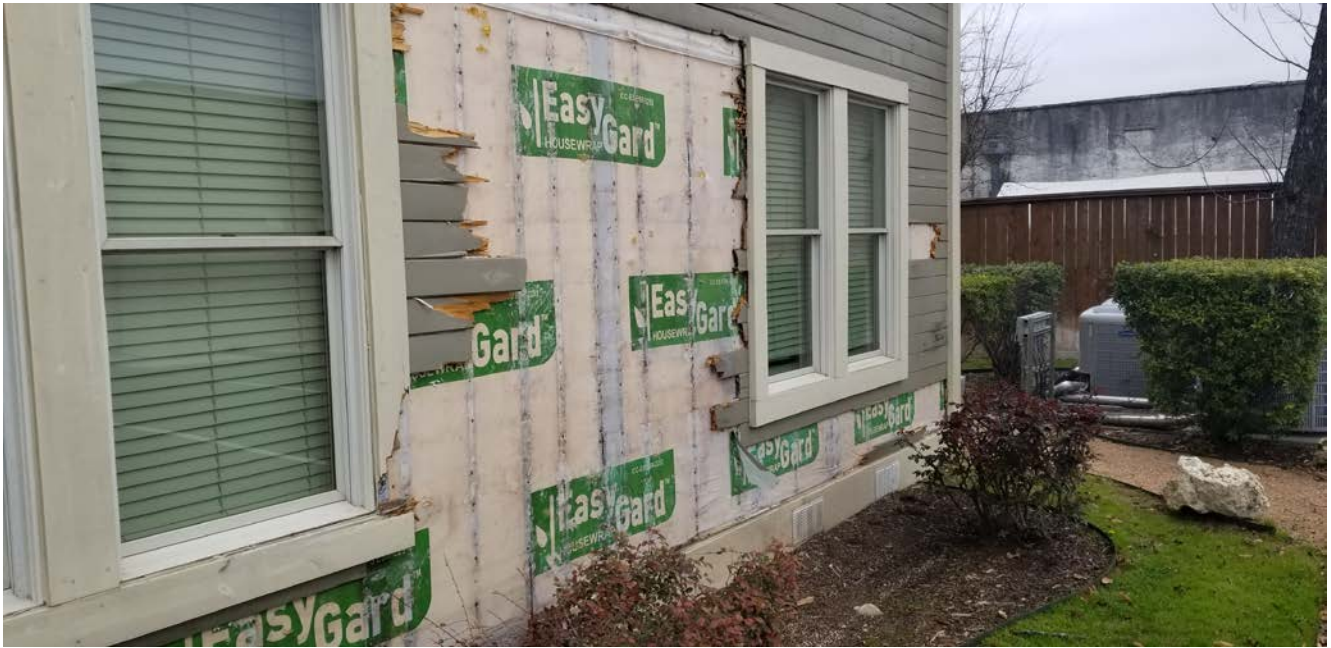
Picture 1: Deteriorated Siding and Trim
