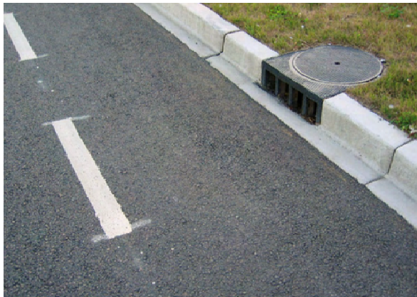
Curb and Gutter
