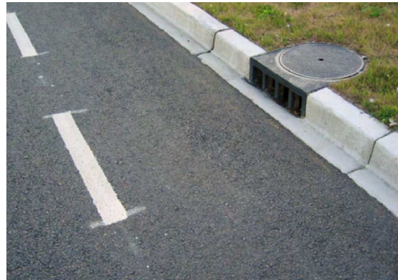
Curb and Gutter
