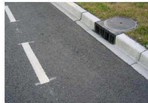
Curb and Gutter
