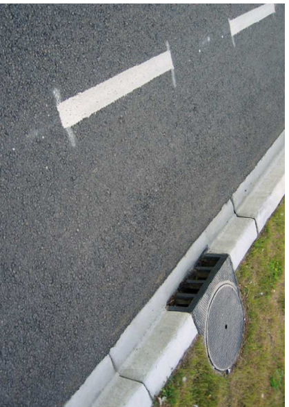
Curb and Gutter
