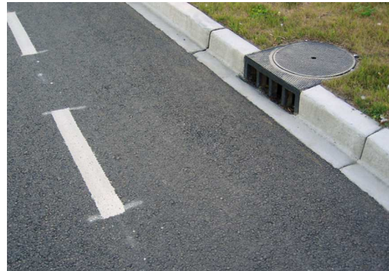
Curb and Gutter
