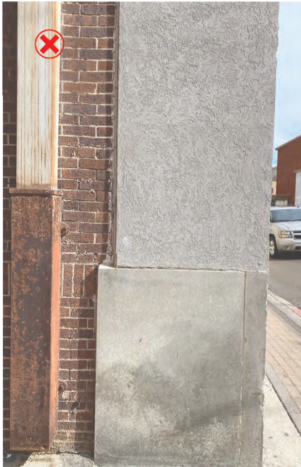
Example of EIFS covering historic limestone. Not appropriate treatment.
