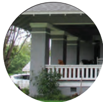
COLUMNS SUPPORTING THE ROOF
