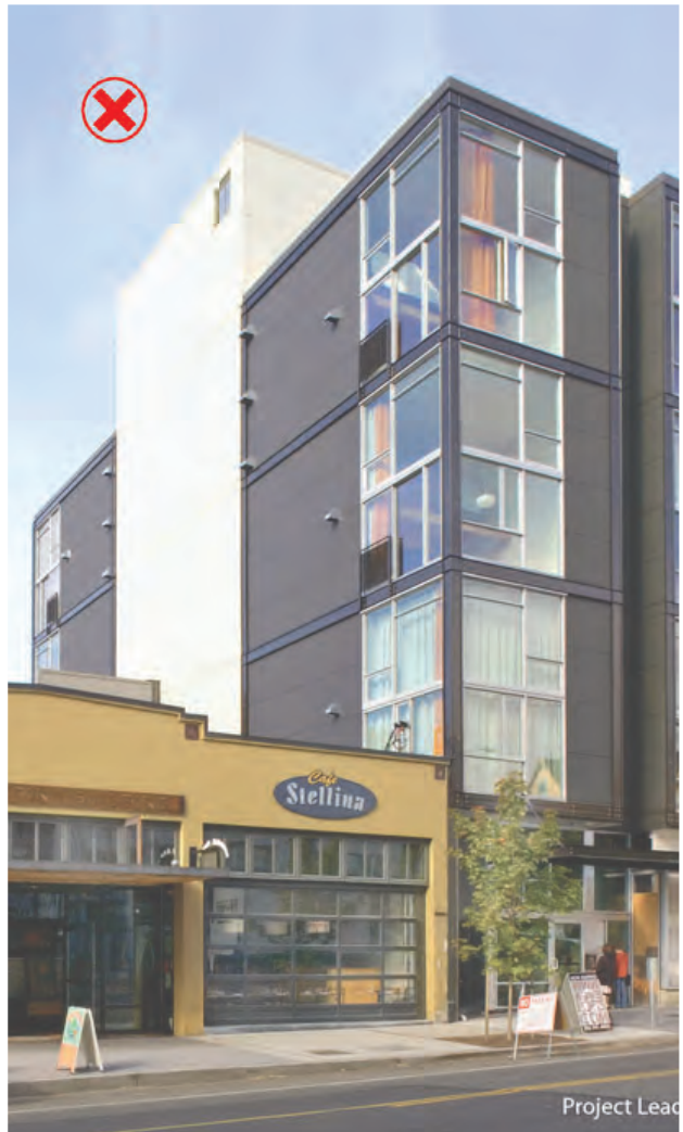
This infill construction is incompatible in massing, scale, and materials.
