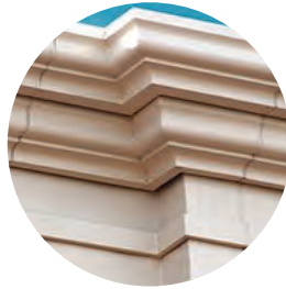
Fiberglass for formed metal, for example in cornices.
