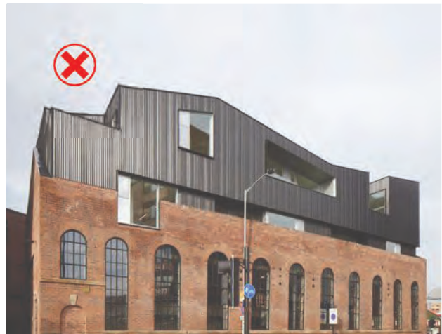
This addition is not compatible in massing or material. it is out of scale with the historic building.
