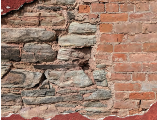
Historic masonry with deteriorated stucco.
