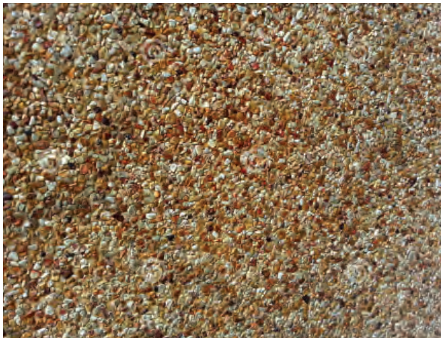
Exposed aggregate detail.
