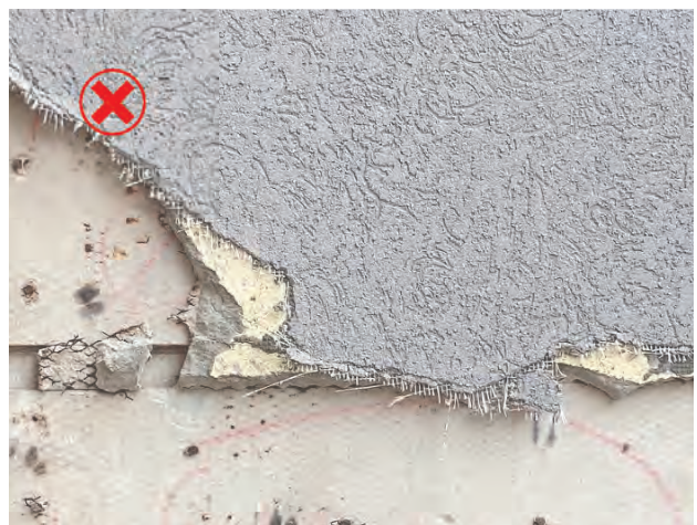
Damaged stucco detail.
